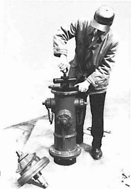
3 Next, attach the Seat Removal Wrench
