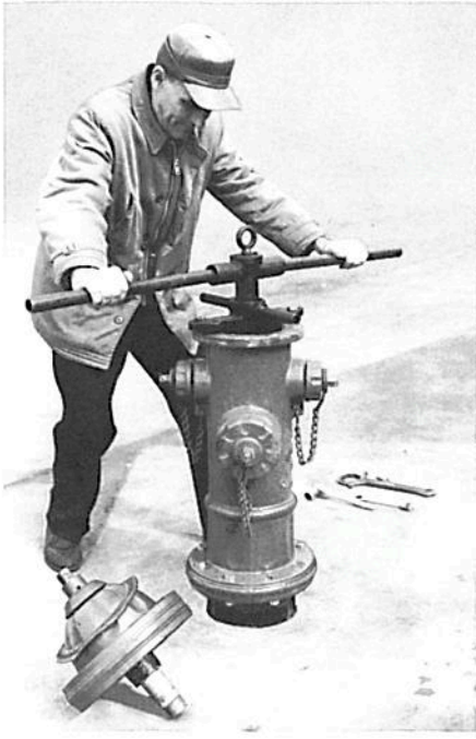
4 Remove main valve and seat ring
