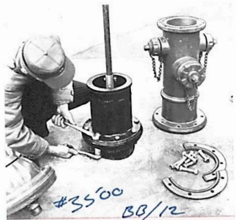
Barrel and stem extensions can be added to raise the hydrant to meet changes in the grade line.
