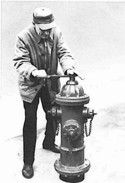
1 First isolate the hydrant
